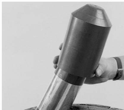
Wipe loose dirt from cable and slip end cap over the cable
