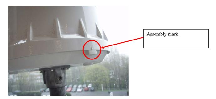
Twist the radome top approx 30 deg. Clockwise. Finally secure the radome with the three set screws.
