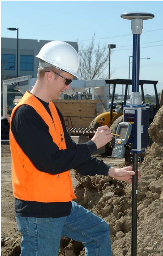
Figure 4.9 Pole-Mounted Rover System Ready to Survey
