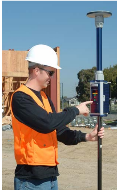
Figure 3.6 Pole-Mounted Rover Setup
