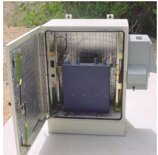
RS 8600 in the central office video head-end and RS 3000 in field cabinet installations
