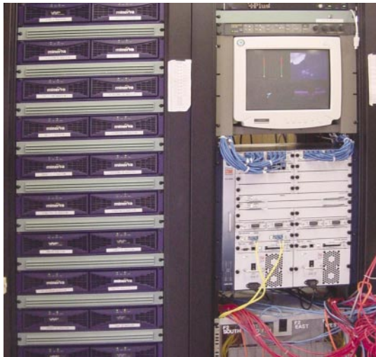
RS 8600 in the central office video head-end and RS 3000 in field cabinet installations
