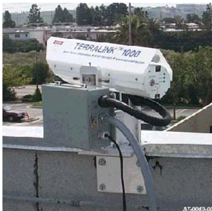
Figure 10: Angle Bracket Mount (M001)
