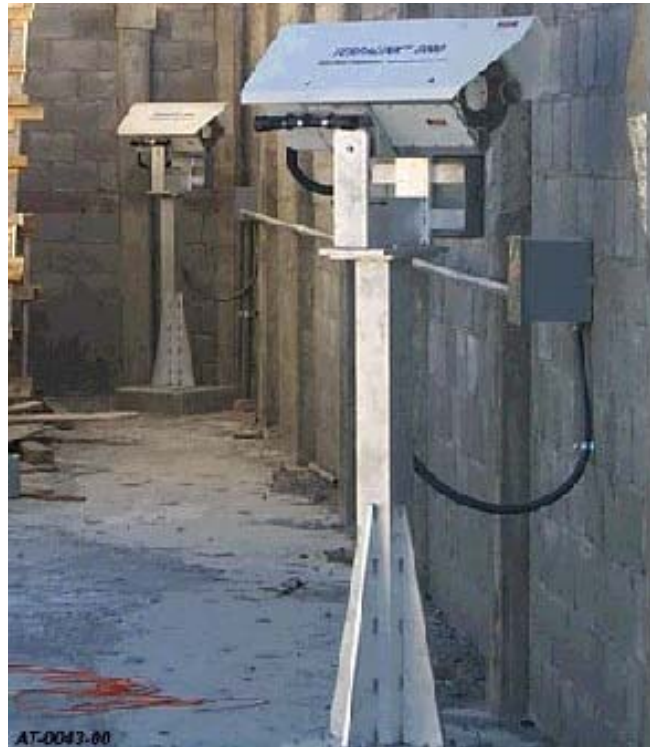
Figure 11: Floor Pedestal Mount (M015)
