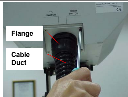
Disconnecting the flange and cable duct – close-up view
