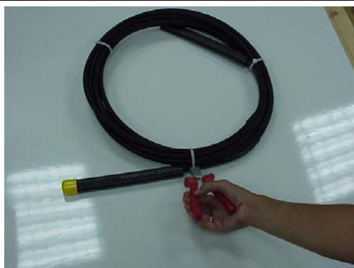
Cutting off the plastic bands of the fiberoptic cable.
