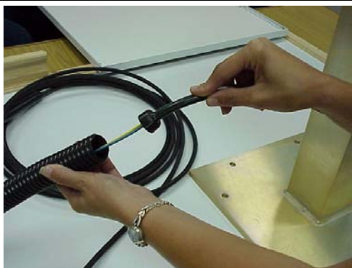
Slipping the fiberoptic cable through the duct and flange.
