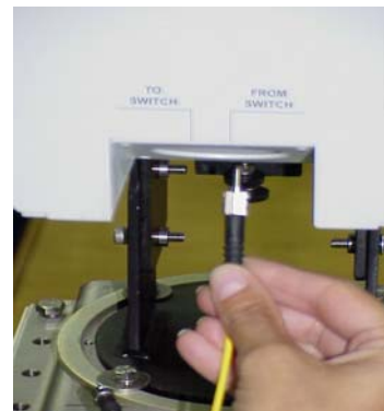
Connecting the other end of the Transmit fiber to the FROM SWITCH port on the TereScope 1 transceiver.
