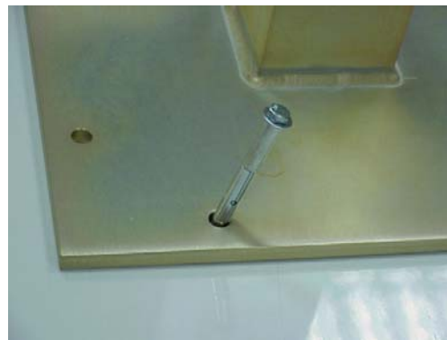
Inserting Concrete Bolts.
