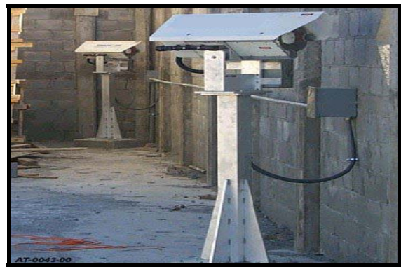
Figure 11: Floor Pedestal Mounting (using JMP and M015C)
