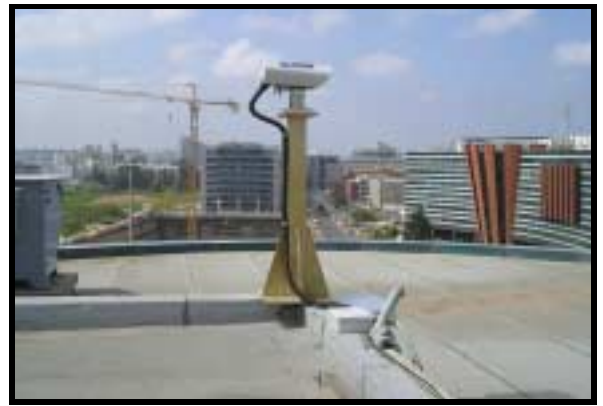
Figure 2.7: Floor Pedestal Mounting (using JMP-L and M015C)
