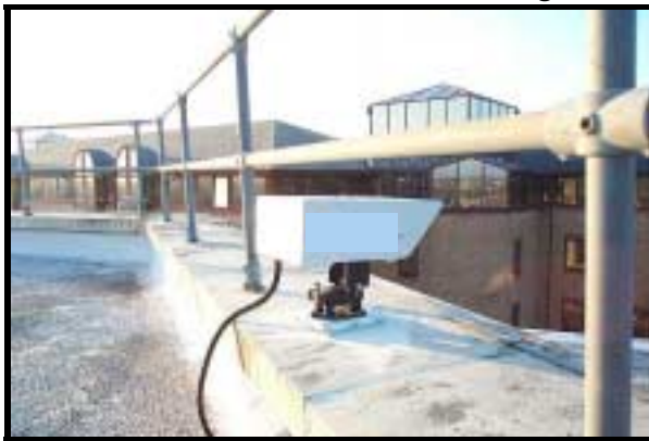
Figure 2.6: Parapet/Ledge Mounting (using JMP-L only)
