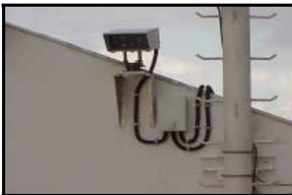
Figure 2.8: Wall Mounting (using JMP-L and JMB)
