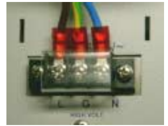
Fig. 6.4: Power cable & Terminal block Fig. 6.5: Power Terminal Block Locked
