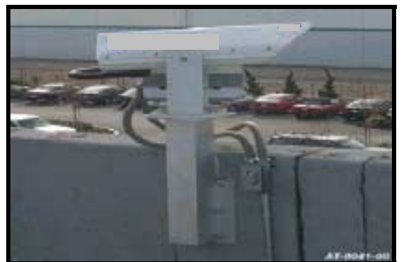
Figure 2.9: Wall Pedestal Mounting (using JMP-L and M054C)
