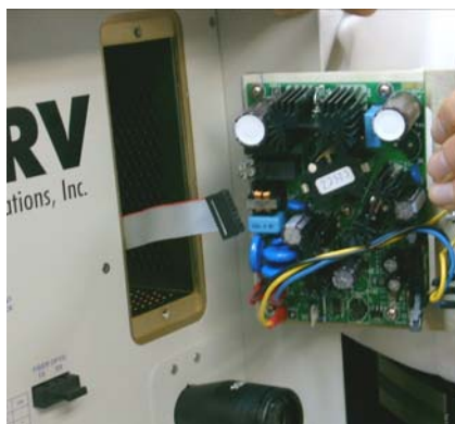
Figure I.3: Disconnected Flat Cable
