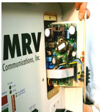
Figure I.2: Pulled out Power Supply
