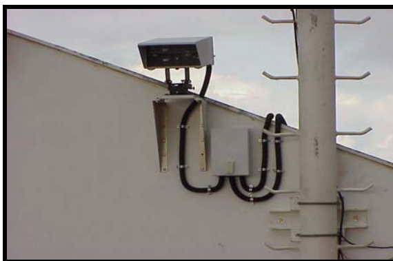
Figure 2.8: Wall Mounting (using JMP and JMB)
