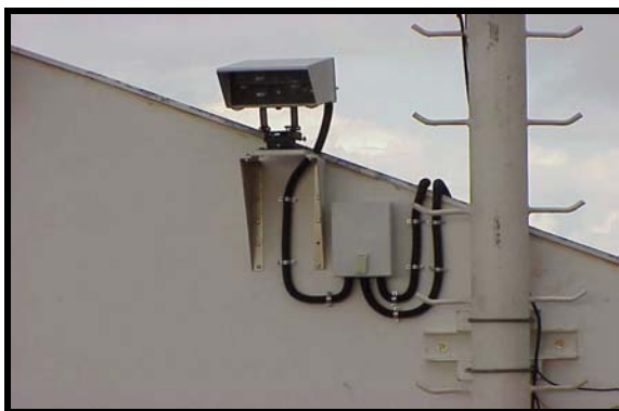
Figure 2.8: Wall Mounting (using JMP and JMB)
