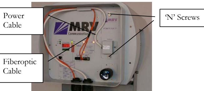
Fig. 6.2: Power cable Fiber optic cable, and 'N' Screws
