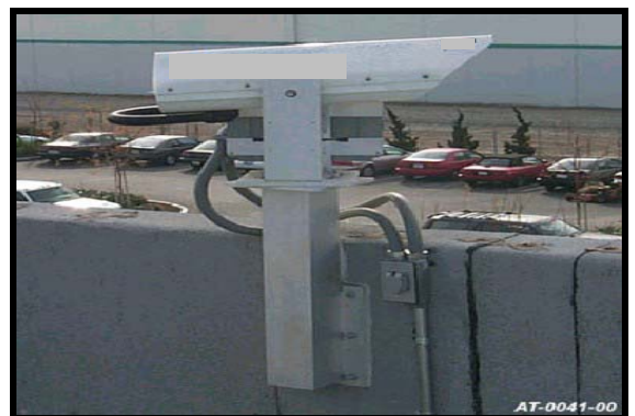
Figure 2.9: Wall Pedestal Mounting (using JMP and M054C)
