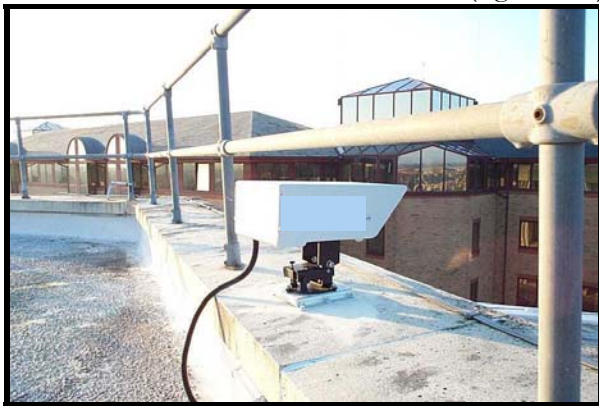
Figure 2.6: Parapet/Ledge Mounting (using JMP only)
