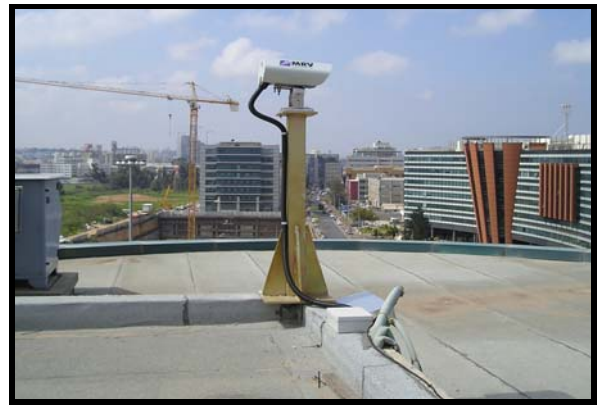
Figure 2.7: Floor Pedestal Mounting (using JMP and M015C)
