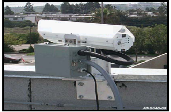
Figure 2.11: Angle Bracket Mounting (using JMP and M001)
