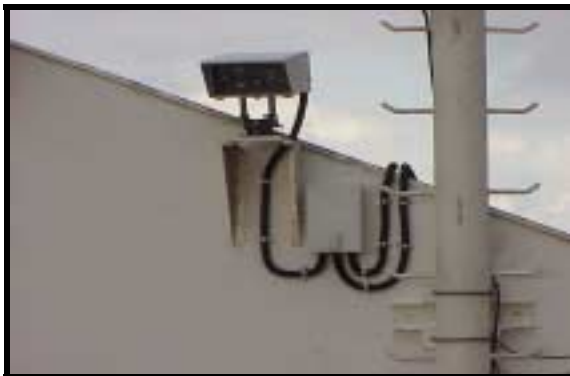
Figure 2.8: Wall Mounting (using JMP and JMB)
