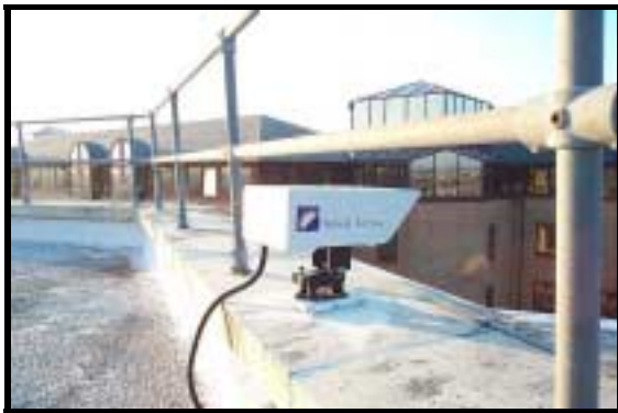
Figure 2.6: Parapet/Ledge Mounting (using JMP only)
