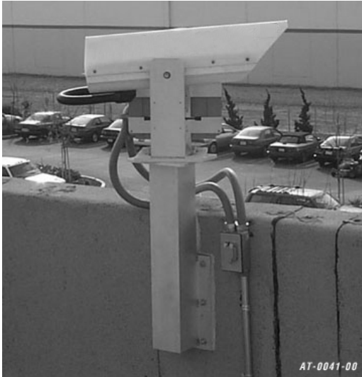
Figure B-3. Wall Pedestal Mount - Used when the link needs to be elevated above the top of a wall.
