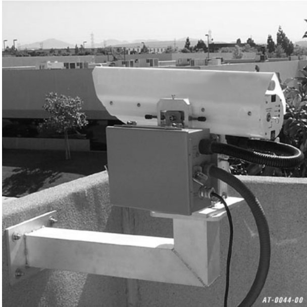
Figure B-6. Extended Wall Mount – Used when a standard wall pedestal mount is insufficient to clear obstacles or for applications requiring an extension from the wall for better access to the transceiver.
