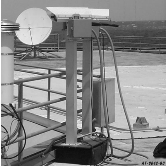
Figure B-4. Floor Pedestal Mount - Similar to the Wall Pedestal Mount.
