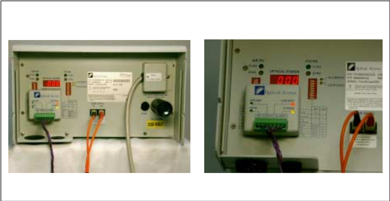
Figure 3. Installation of the dry contact expansion module
