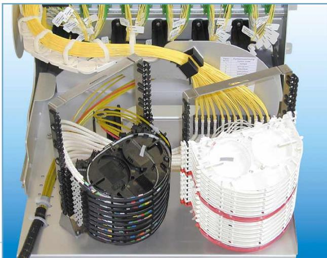
VIP Distribution Frame from rear with 10 black inline splice trays on left and 2 red distribution trays combined with 6 white subscriber trays on the right
