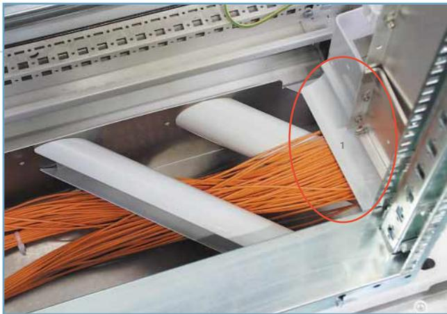
*Bottom Section Installed, with Horizontal Division (1)*
