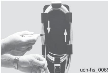
7.3 In the slack storage, route the buffer tubes in an arc and mark the stripping length according to table 1 and sketch 5.
