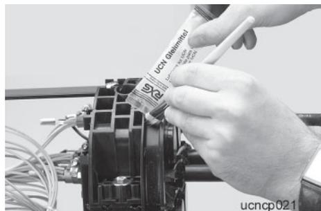
**11.3** Brush sealing slot of the end cap thinly with lubricant.
