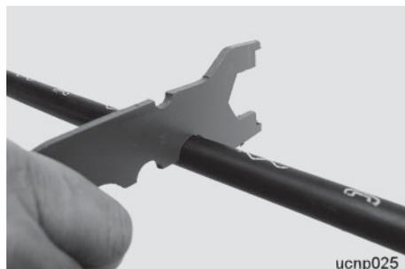
6.3 Clean cable end. Remove printing in sealing area by scraping with back of knife. Use gauge to determine which sealing is required.
